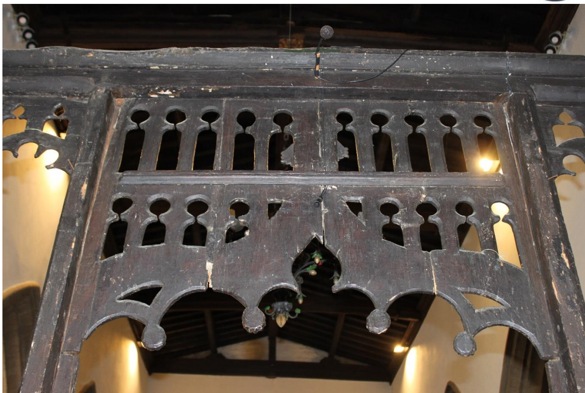
Plate 7: View to the chancel facing side of the decorative central arch of the screen from the chancel, looking west (Credit: Esther Robinson Wild)
