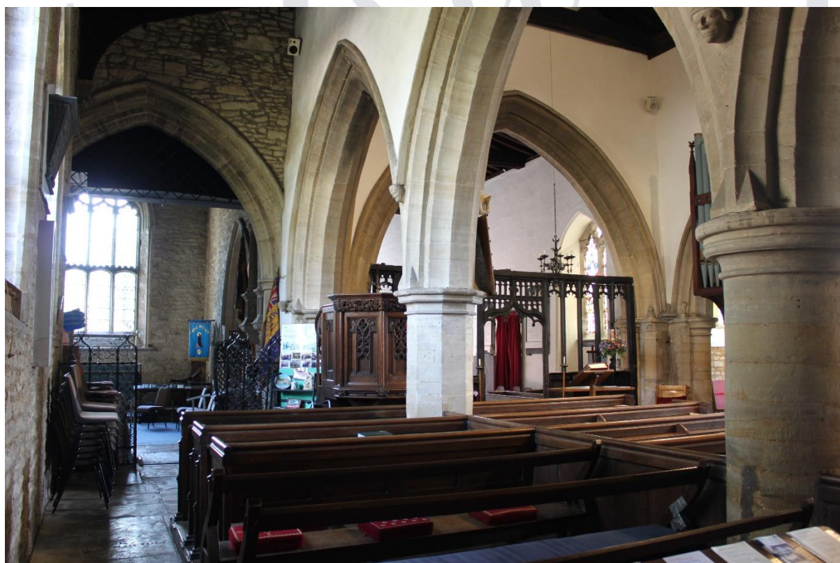
Plate 4: View to the Tofte Chapel, pulpit, nave facing side of the screen and the chancel from the north aisle, looking southeast (Credit: Esther Robinson Wild)
