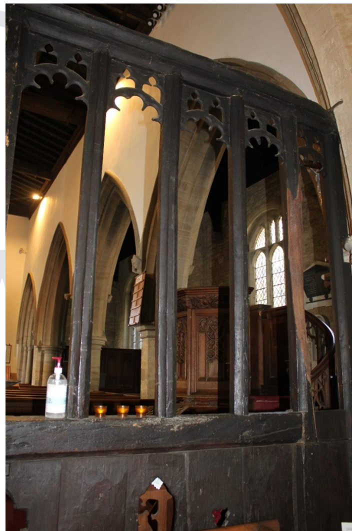
Plate 19: View to the window lights on the chancel facing side of the north side of the screen from the chancel, looking northwest (Credit: Esther Robinson Wild)
