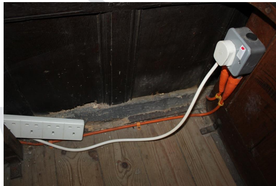
Plate 23: View to a section of sill on the chancel facing side of the north side of the screen from the chancel, looking northwest (Credit: Esther Robinson Wil)
