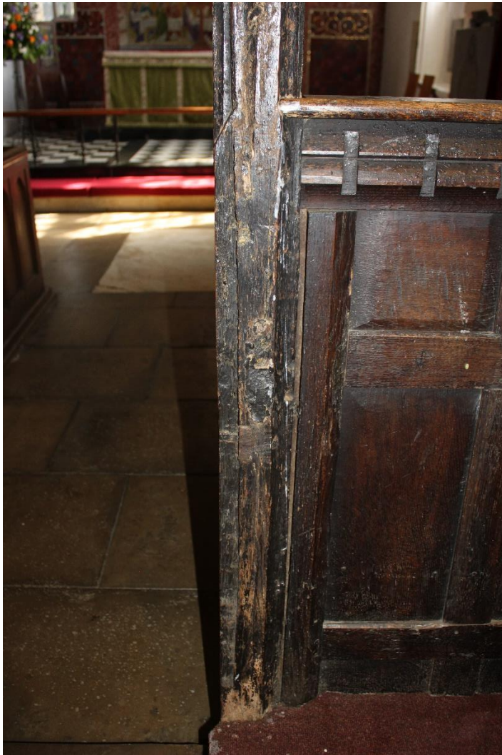
Plate 14: View to the post of the south side of the screen from the nave, looking east (Credit: Esther Robinson Wild)
