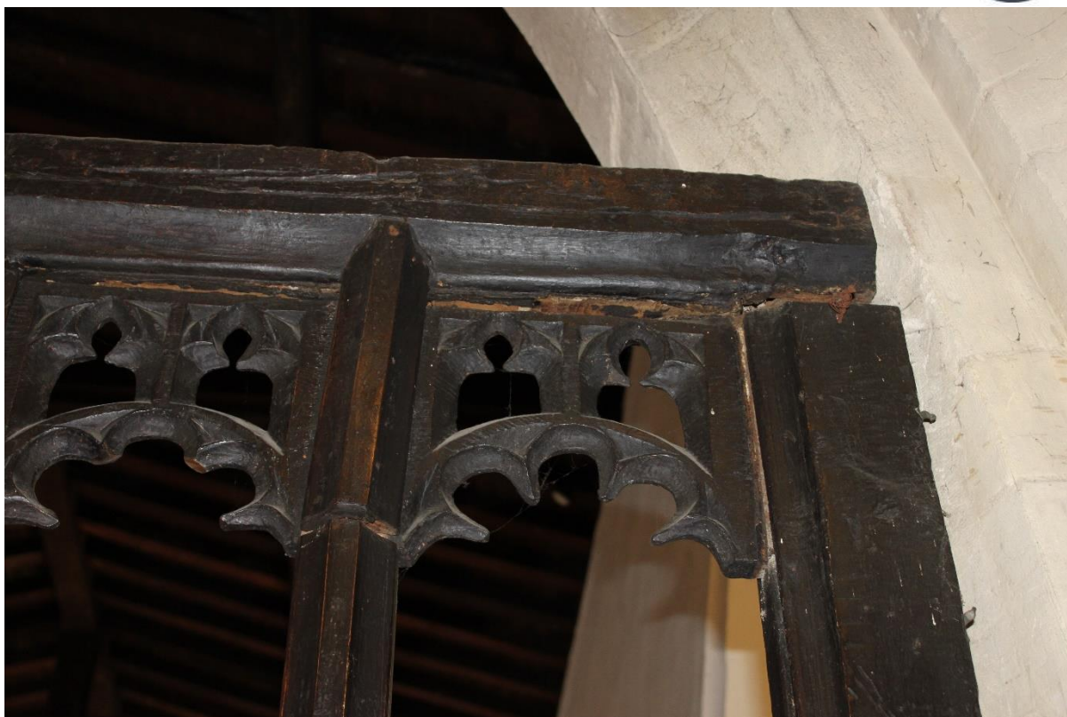
Plate 12: View to top of the window lights of the south side of the screen from the nave, looking east (Credit: Esther Robinson Wild)
