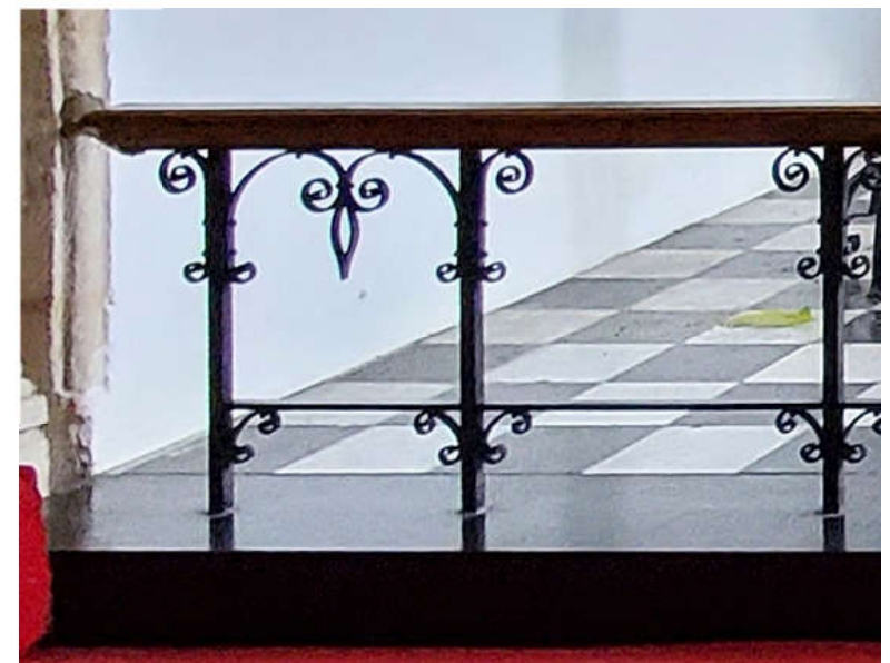
Existing Altar Rail
