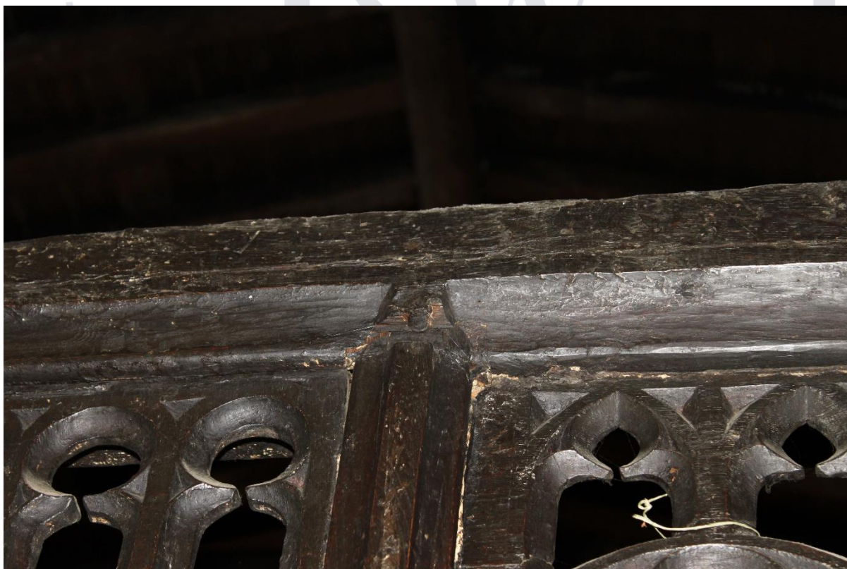
Plate 13: View to the top of the window lights (and metal nail) of the south side of the screen from the nave, looking east (Credit: Esther Robinson Wild)
