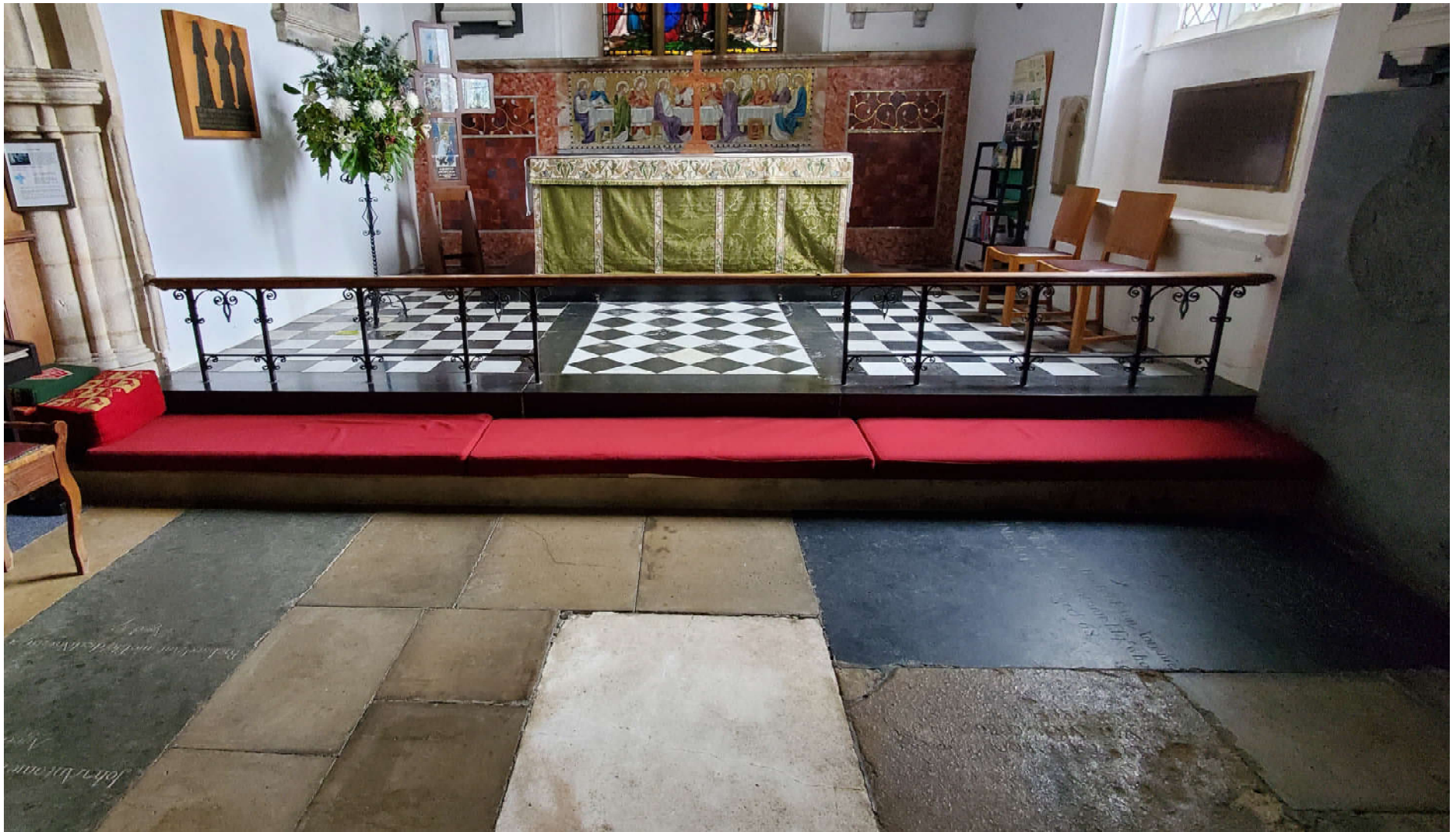
Existing Altar Rail.
