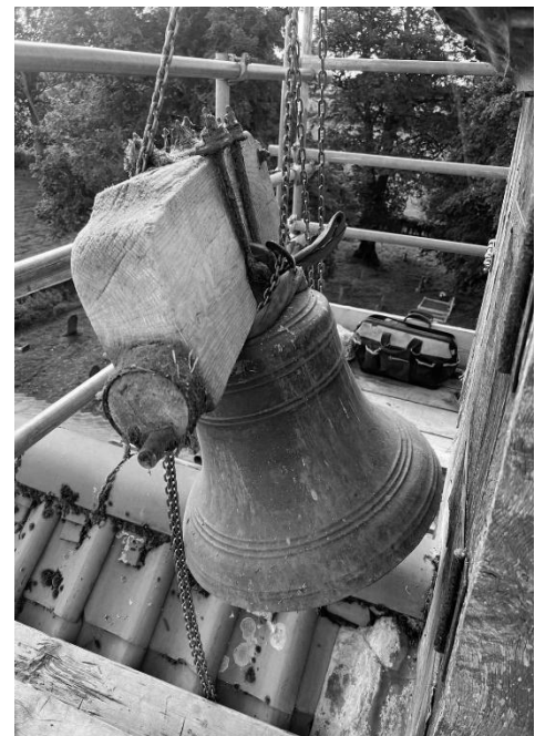
The bell being removed for renovation in September 2025
