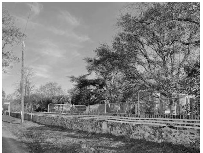
The finished repaired wall
