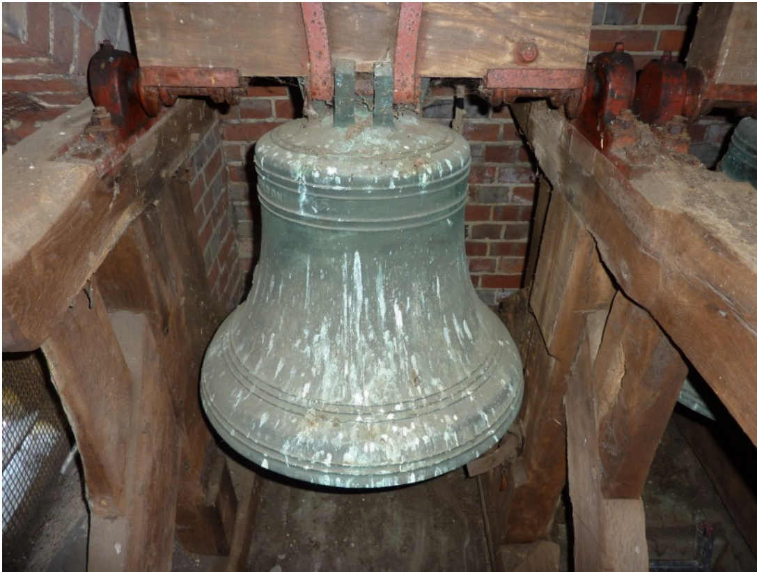
The 3 rd or Tenor Bell, now rung by an electric hammer. This bell is now controlled by a timer device and strikes the hour, as if it were a clock!
