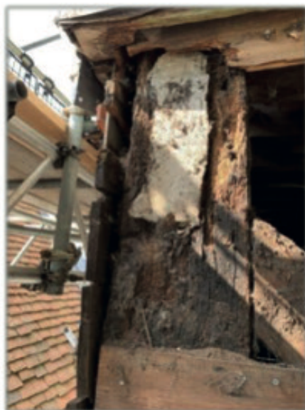
Damp damage to main corner support of ringing chamber showing concrete infill from previous repair
