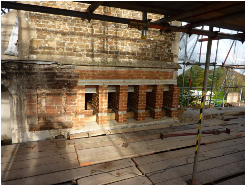
Left: December 2011, underpinning the leaning Victorian tower
