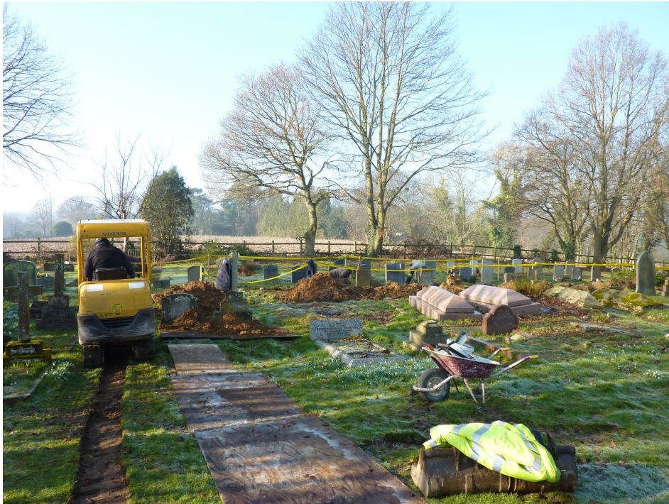
Left: Excavations in the churchyard to lay gas and water pipes February 2013
