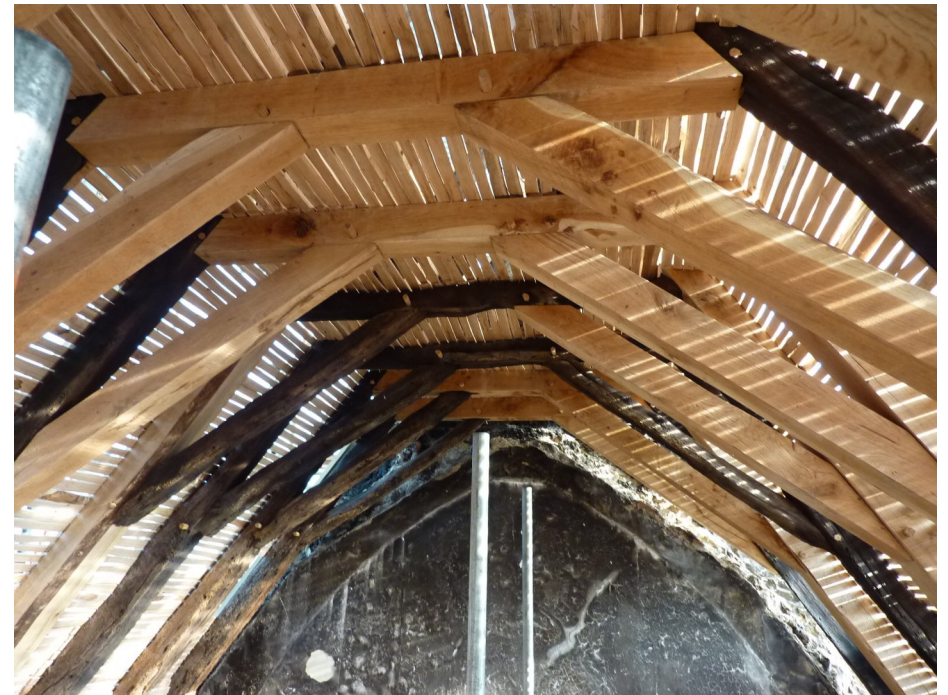
Oct. / Nov. 2011 and the timbers start to go back, 80% are original
