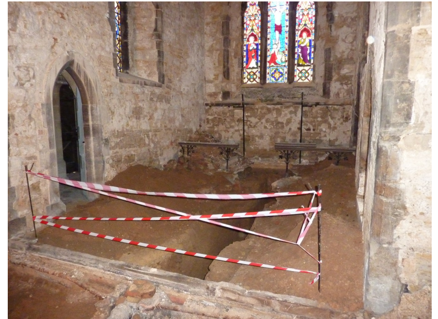
Left: December 2011, underpinning the leaning Victorian tower
