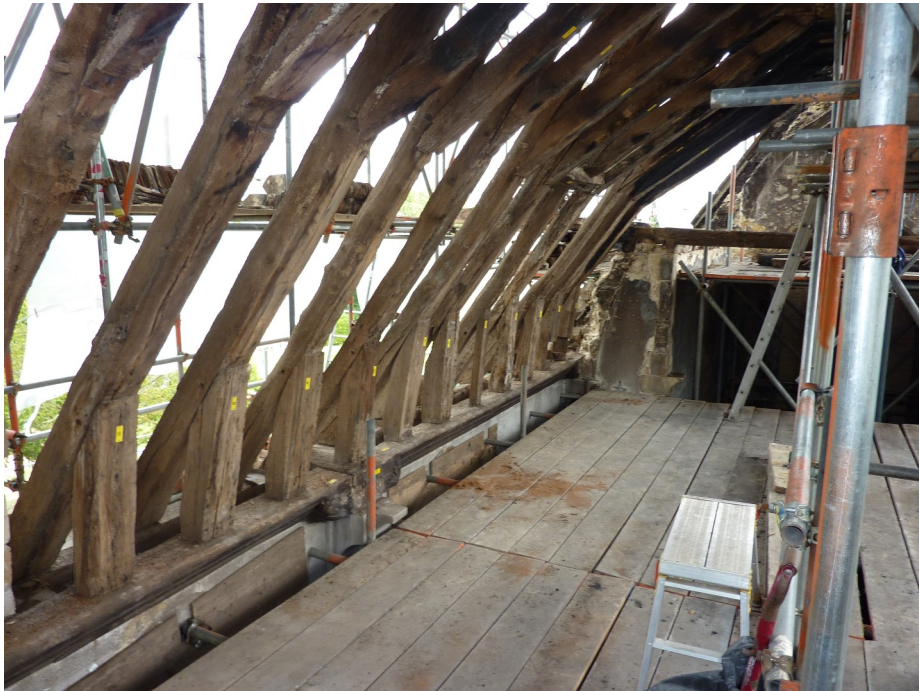
Oct. / Nov. 2011 and the timbers start to go back, 80% are original
