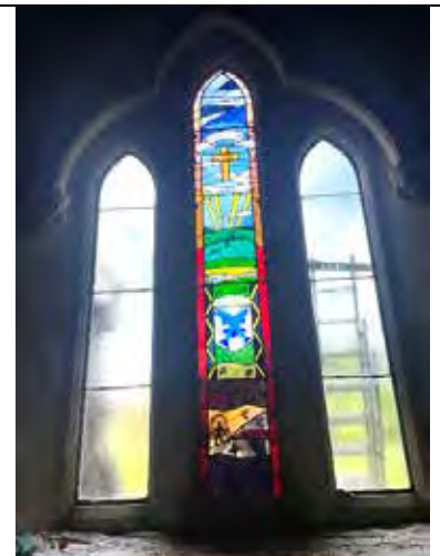
Figure 7 The middle light (Ch.2) is installed. The ladder is positioned to carry on with Ch.3.
