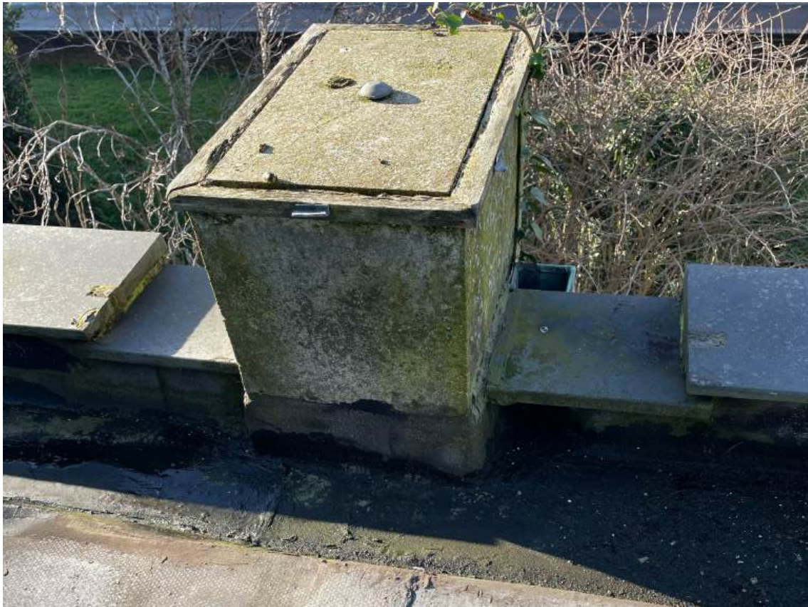
View of pier missing its capping and hopper and downpipe South aisle roof St Andrew and St George
