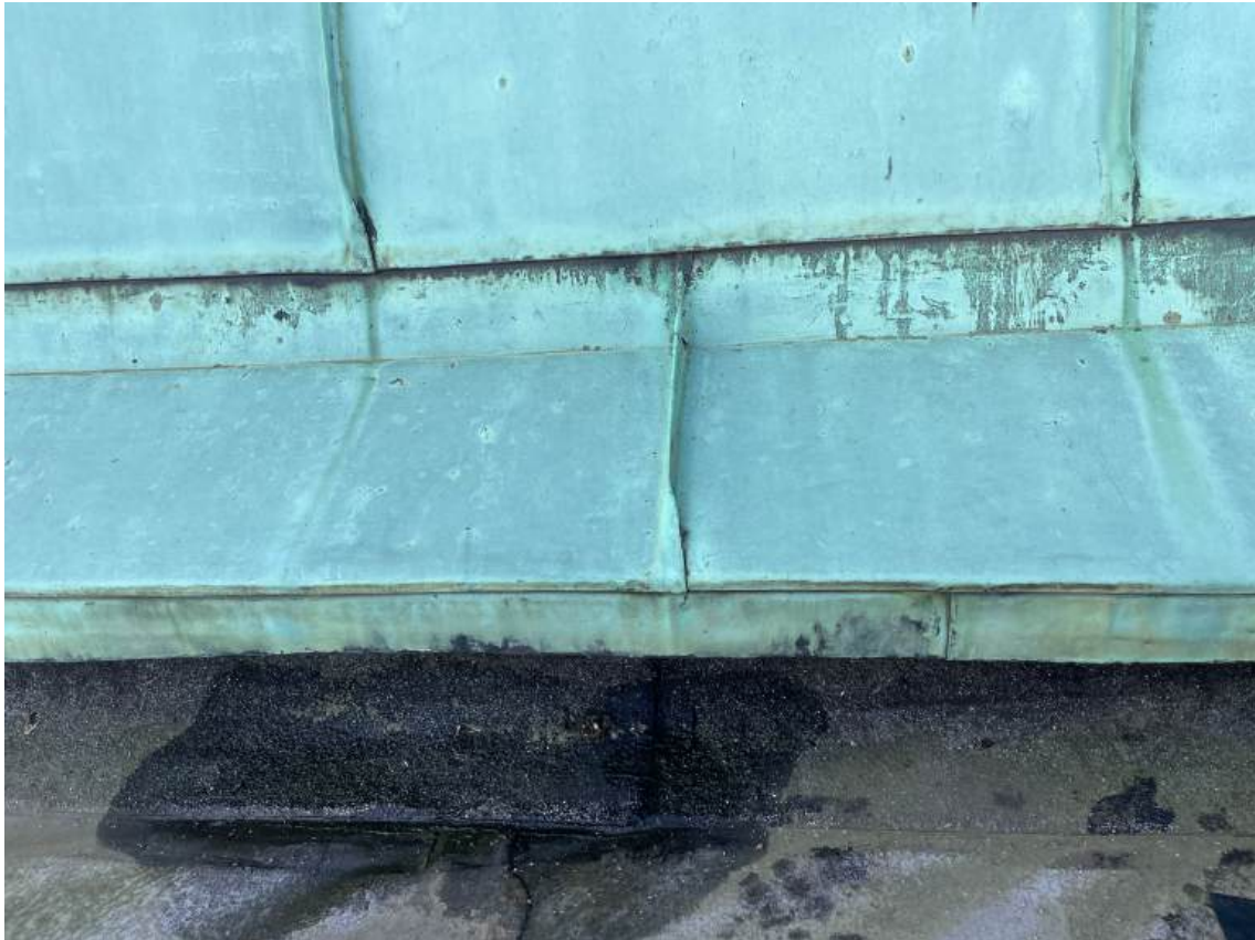
View of upstand and drip flashing to copper half barrel South aisle roof St Andrew and St George
