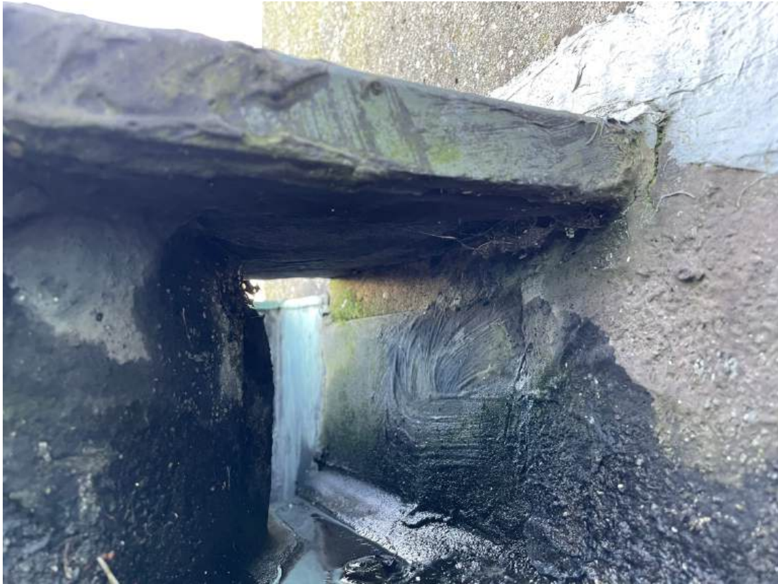
View of scupper through parapet South aisle roof St Andrew and St George
