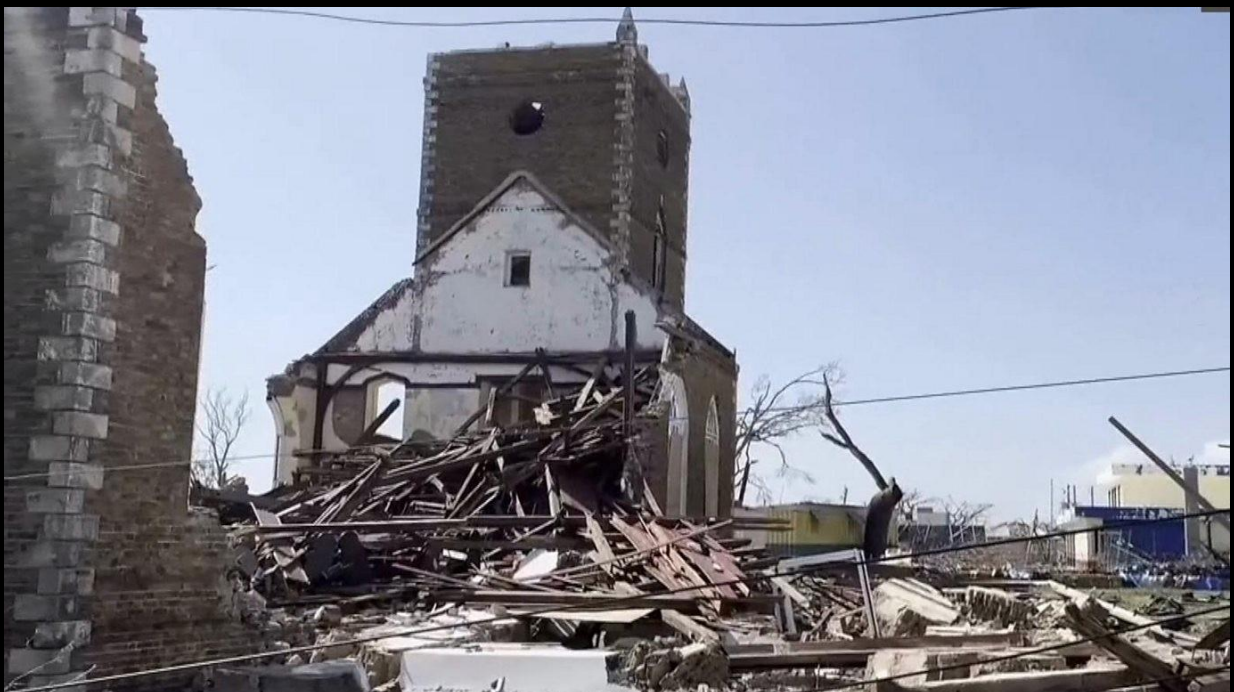
The destruction Hurricane Melissa caused to St John's Anglican church, a 300-year-old church this week
