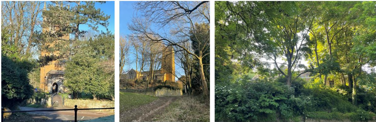
Figure 1: Views of the church (L) from the south, and (centre and R) from the northwest showing its position on the Jurassic ridge, in winter and summer (the rise on the left contains the C19 cart wash / pond).
