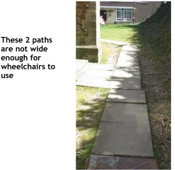
Path on South side at east end. Trip hazards on uneven paving
