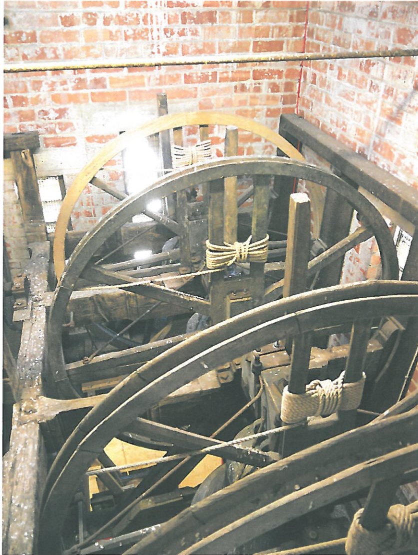
Detail of bell frame.
