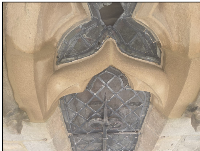
New carved tracery stones around the windows replaced weathered stone. Glazing was also repaired.
