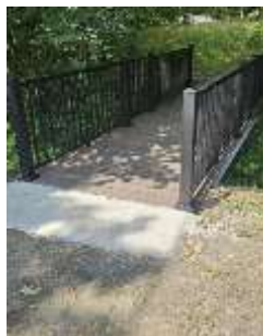
New bridge over the stream for the quiet garden.
