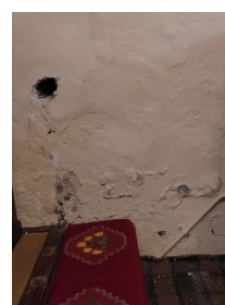
Damp in the vestry and near the altar
