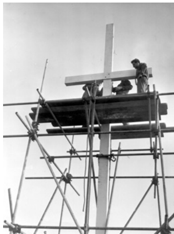
Installation of the cross from HMS Ganges
