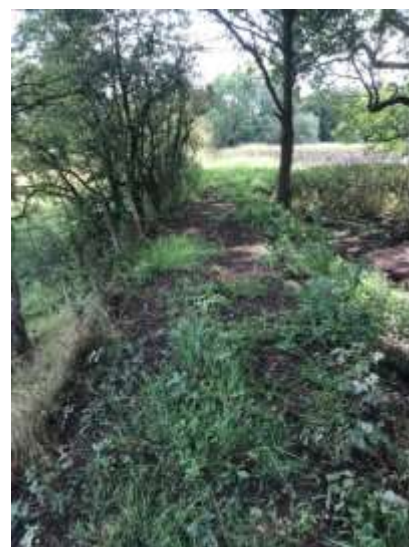
Top end AFTER construction
