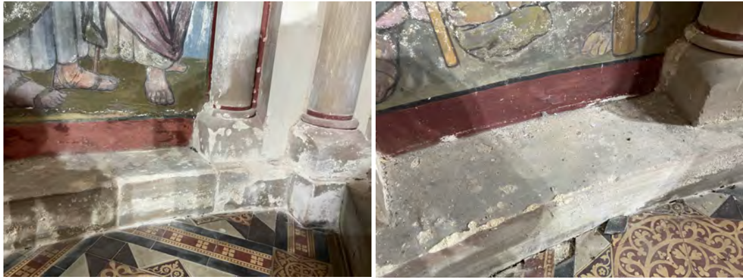
Detail of the condition of the surrounding stone, Ss Bartholomew and Philip, left. Right, spalling surrounding stonework, Ss James Major and Thaddaeus, as well as fragments of the painted surface on the stone step
