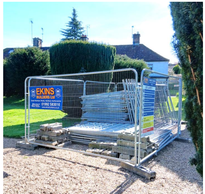
Photo: Fencing has already arrived on site
