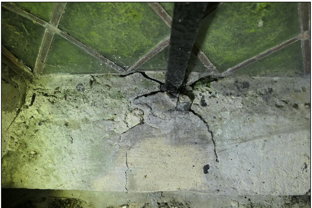
Fig.5 – Rusted and expanded stanchion now jacking open the sill. Thick green layers of algae on both faces of the glass, window wI, interior.
