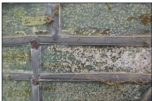
Fig.6 - Dirt and corrosion products collected in surface pits, ext. of B1
