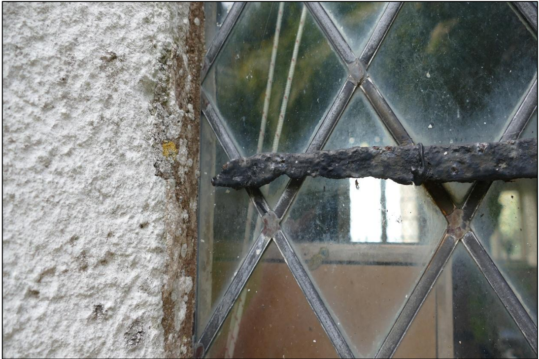
Fig.4 – Medieval lug bar tip completely rusted through and lost, window sV, exterior.
