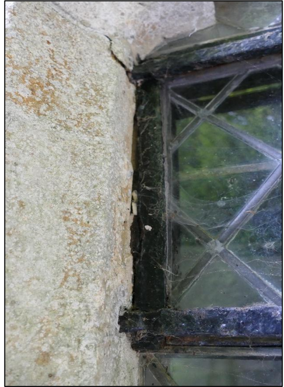
Fig.2 – Masonry joint cracked from inside through to outside due to rusting casement, window sIII, exterior a/b
