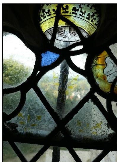
Fig.18 – Faded and lost glass paint on painted quarries, int. face, 2a.
