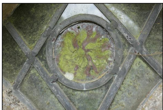
Fig. 7 - Thick, obscuring and potentially damaging layer of algae on glass, ext. of C1
