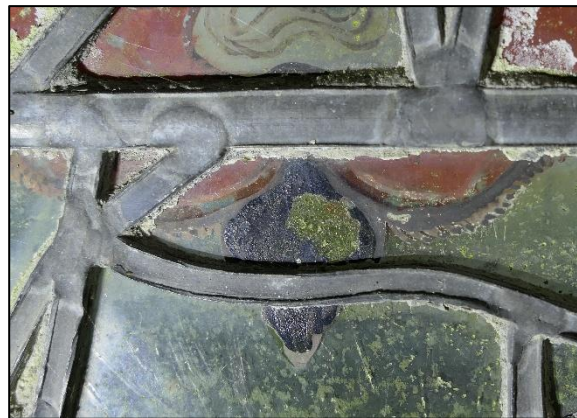
Fig.11 – Blue enamel on rose leaf (silver stain on reverse to make green colour) flaked away and damaged glass surface beneath, int. panel 1b.
