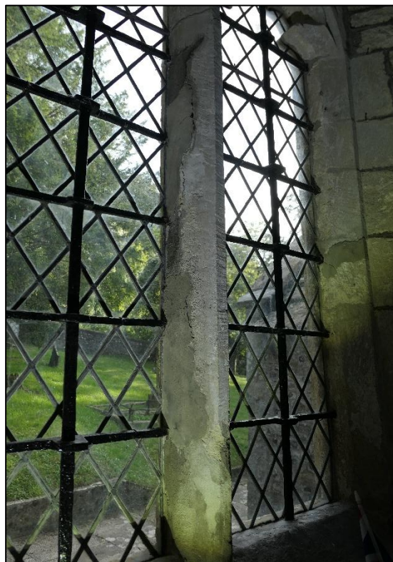
Fig.3 – Several failed mortar repairs to spalled mullion, window sIV, interior.
