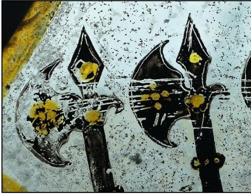
Fig.15 – Scratched and flaking glass paint on pitted interior surface, int. 1c.
