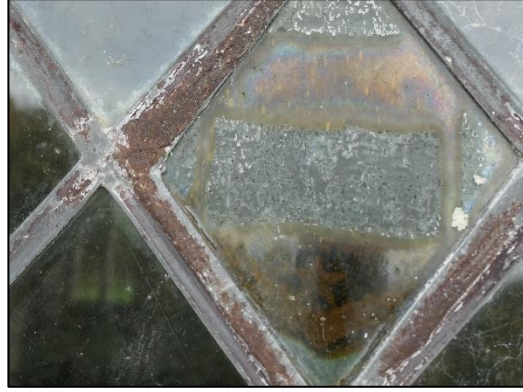
Fig.16 – Reddish corrosion products on ext. lead comes, ext. 1a.
