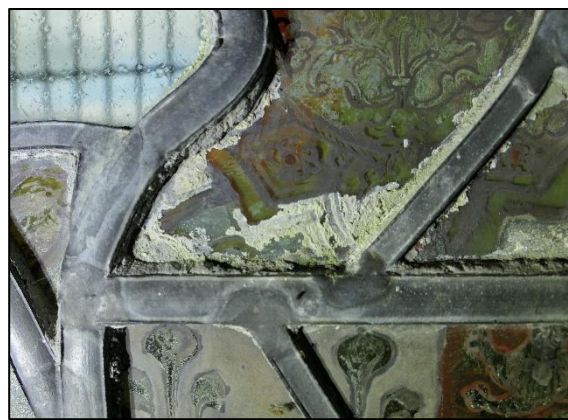
Fig.13 – Calcium carbonate deposits on glass leached from leaded-light cement under lead flanges, int. 1a.
