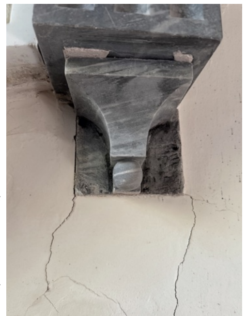
Figure 33 ~ Details of ferrous staining on both sides of the moulding supporting the pediment of monument 5, from corroding iron fixings behind.
