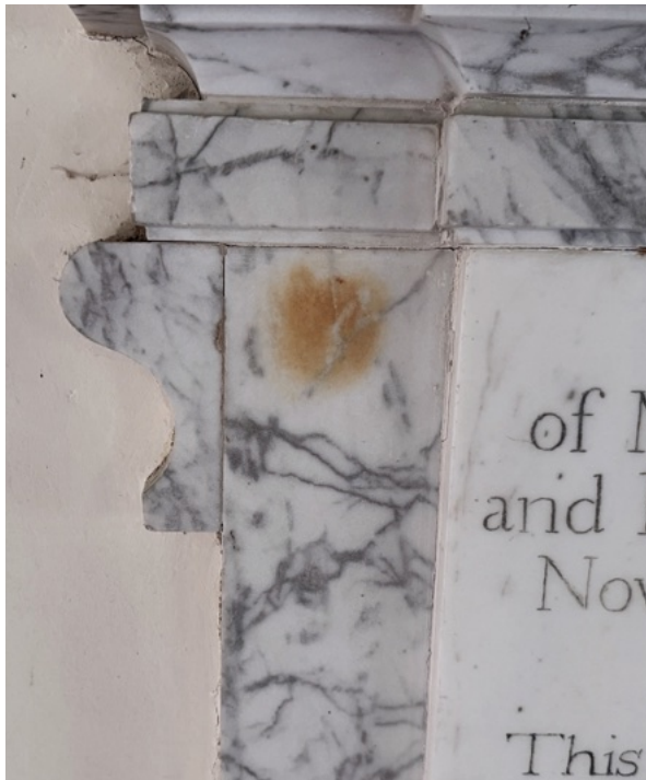
Figure 22 ~ Detail of iron stain on surround of the dexter of monument 001.
