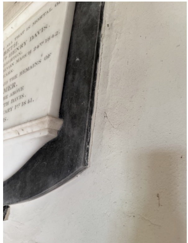
Figure 38 ~ Detail of minor crack around the perimeter of monument 6 on the sinister side.
