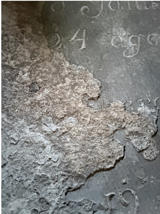
Figure 48 ~ Detail of laminating surface area on inscription of ledger stone 009.
