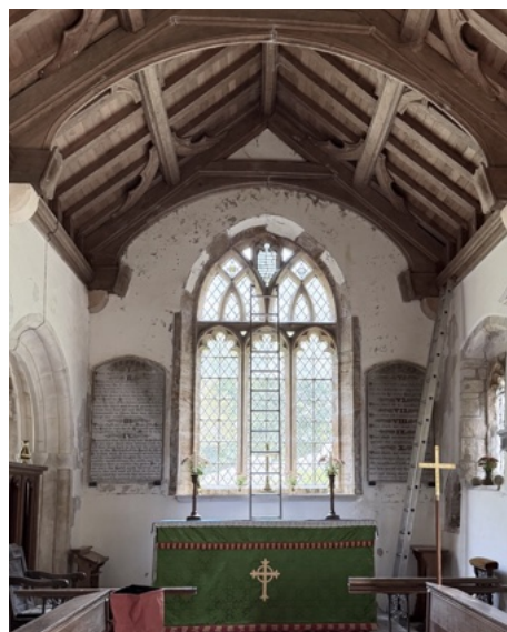
Figure 20 ~ Interior view of the Chancel wall around the Decalogues showing damp.
