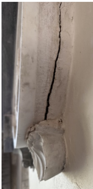
Figure 33 ~ Details of ferrous staining on both sides of the moulding supporting the pediment of monument 5, from corroding iron fixings behind.
