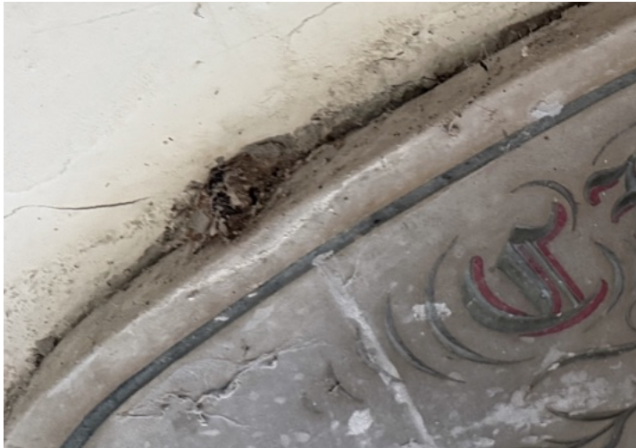
Figure 41 ~ Detail showing corroding iron fixing above Decalogue 1.
