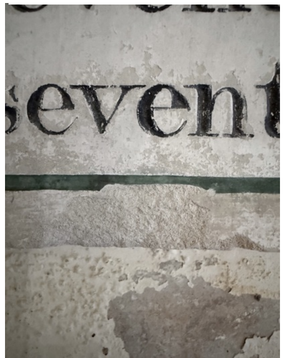
Figure 44 ~ Detail showing loss of stone on decalogue 1.
