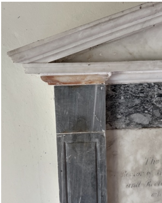
Figure 33 ~ Details of ferrous staining on both sides of the moulding supporting the pediment of monument 5, from corroding iron fixings behind.
