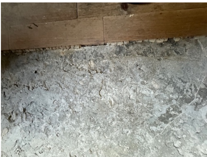
Figure 52 ~ Detail illustrating laminating surface and crumbling mortar around ledger stone 010.
