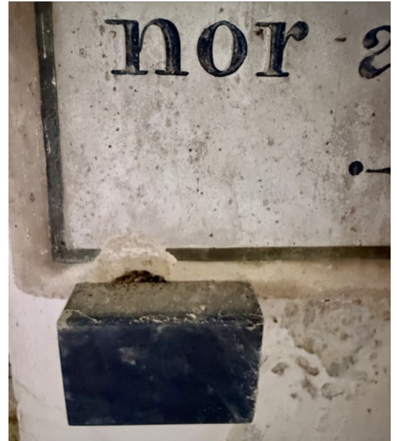
Figure 42 ~ Detail of lower dexter bracket and corroding fixing, Decalogue 1.
