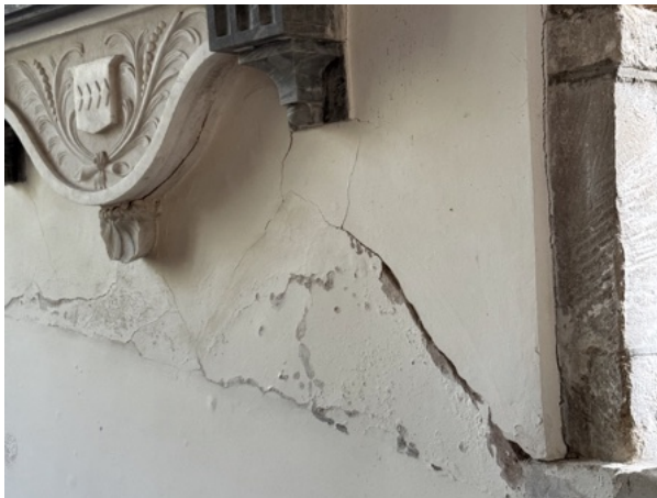
Figure 31 ~ Detail of cracks in the wall around monument 5.
