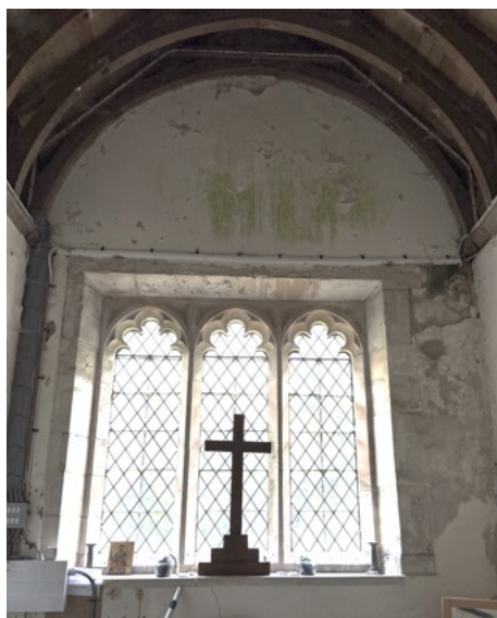
Figure 17 ~ Interior view of the North Chapel showing damp on the east elevation.
