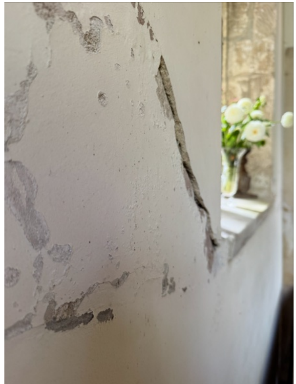
Figure 32 ~ Detail of south elevation beneath the monument, illustrating extensive cracking and movement of wall.
