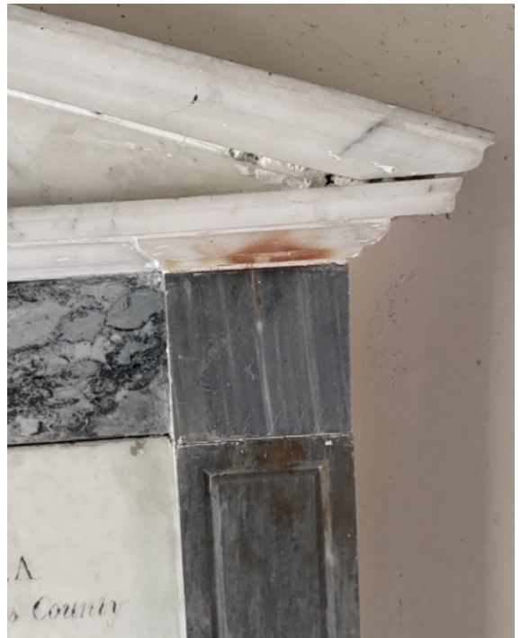
Figure 33 ~ Details of ferrous staining on both sides of the moulding supporting the pediment of monument 5, from corroding iron fixings behind.
