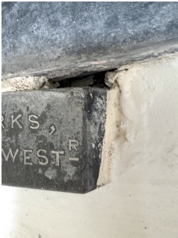
Figure 37 ~ Detail bloomed black surface and minor loss of mortar around the manufacturer's inscription below monument 6.
