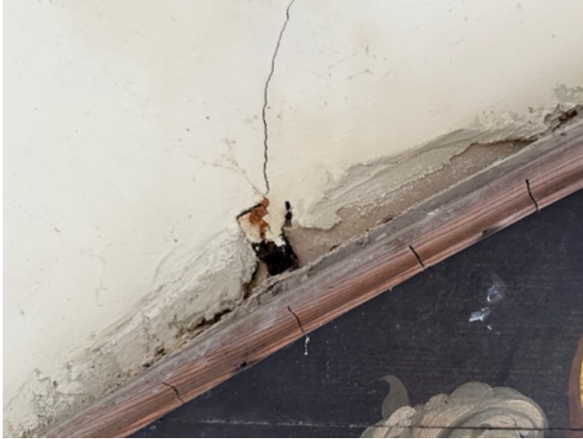
Figure 56 ~ Detail of corroding fixing and frame.
