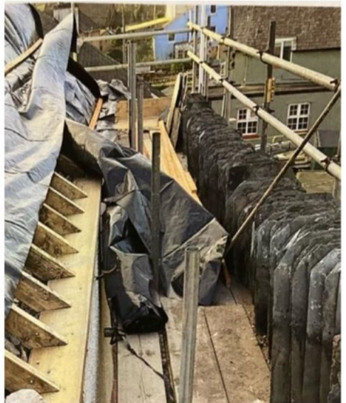
New Roof trusses in place
