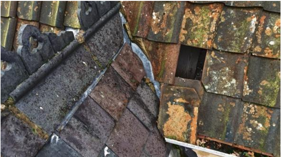
Missing tile on external roof
