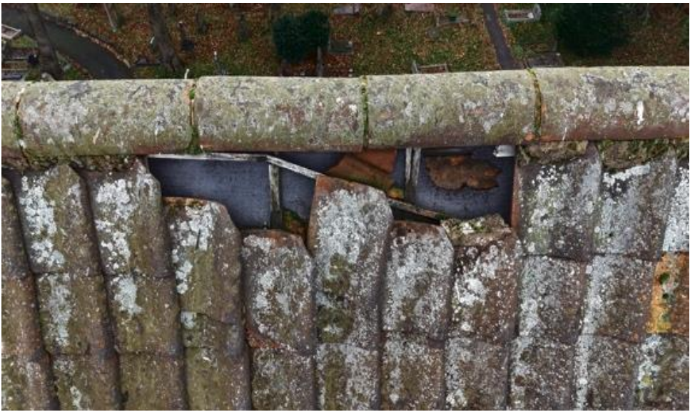
Missing tile and damaged membrane on external roof
