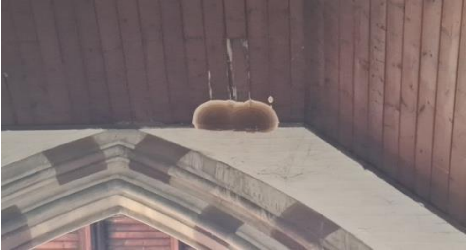
Dry rot on the inside of the roof
