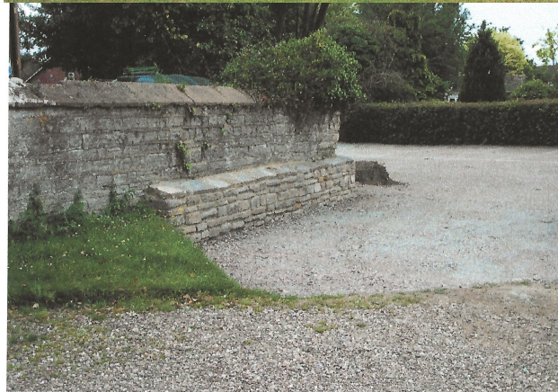
CAR PARK COMPLETED JULY 2011
