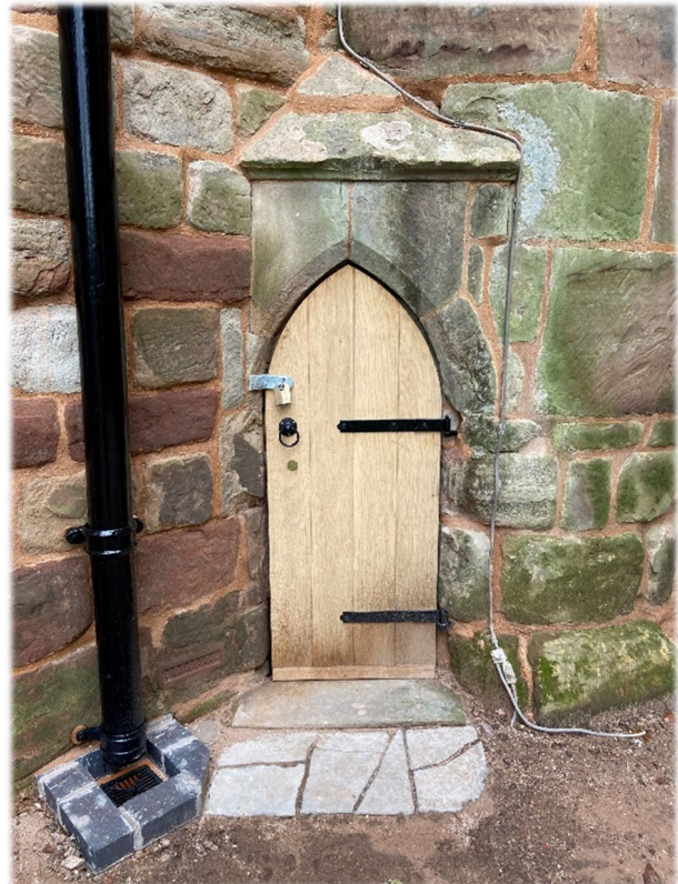
New door now in situ and lime mortar repointing.
