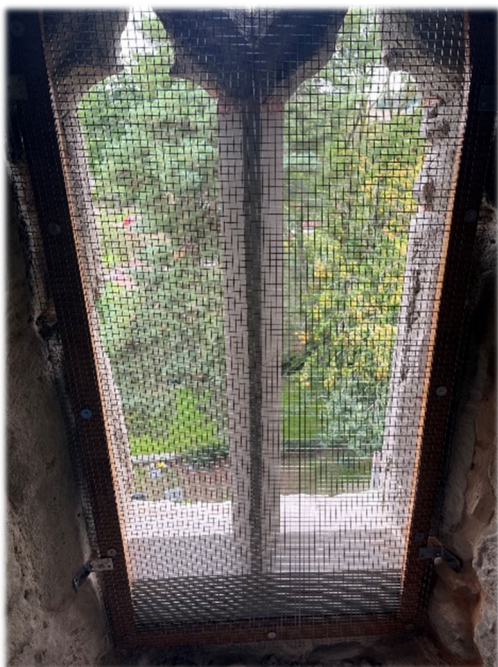
Vertical turret window being fitted with new cill and framing already in place.
