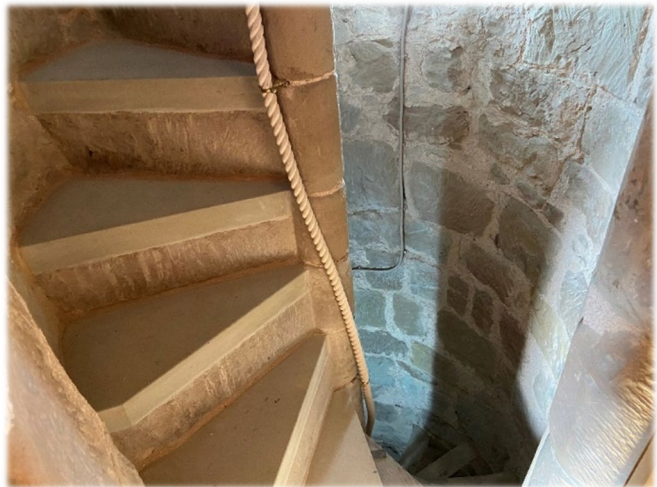
New rope handrail fitted
