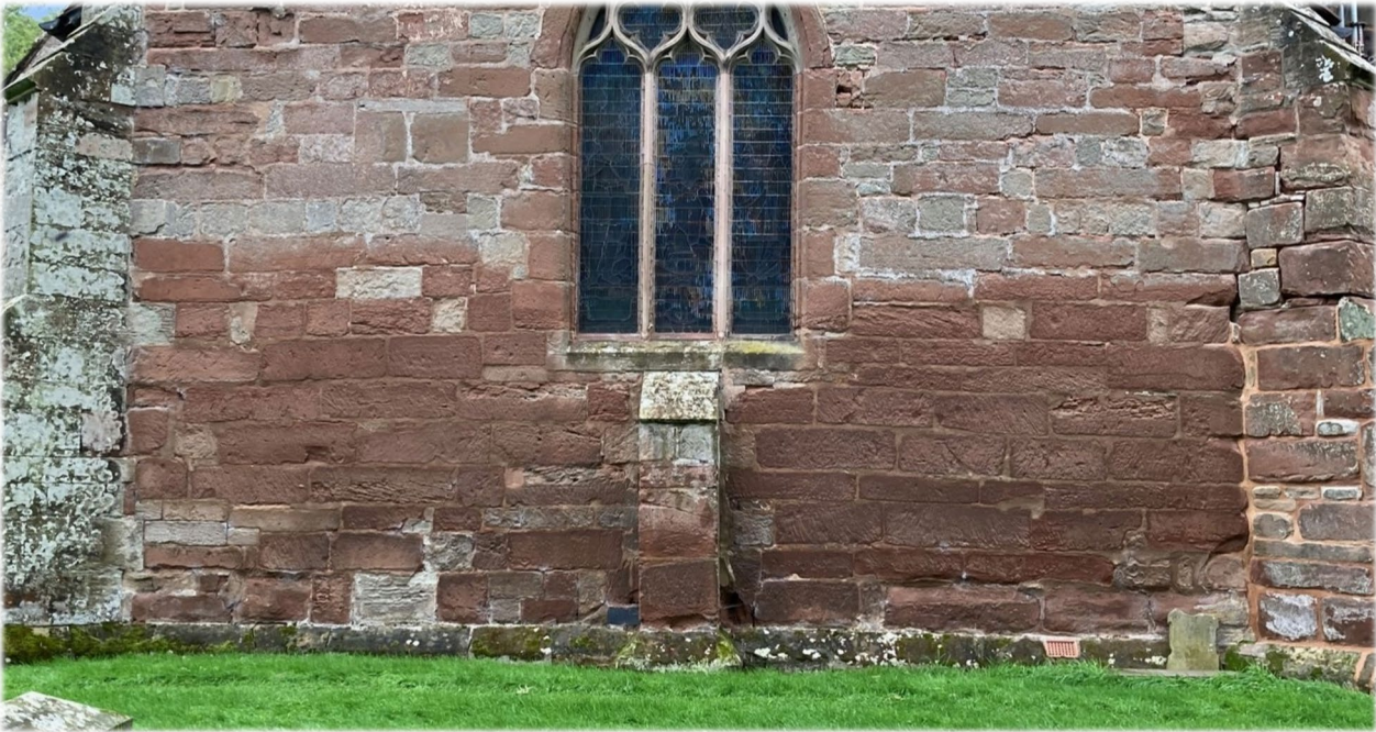
Nave west gable end – stonework pre-project showing cement-base mortar and damp areas.
