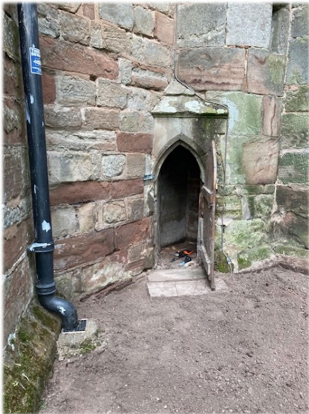
Pre-project: external turret access door cement-based mortar in poor condition, causing damp and damage to stonework.
