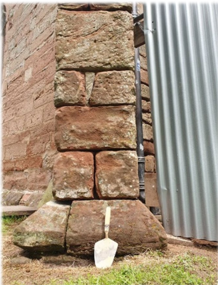
Example of damaging cement-based mortar raked out ready for repointing.
