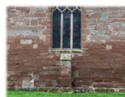
Pre-project cement-based mortar causing dampness
