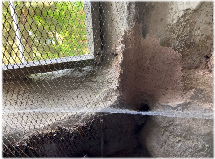
Pre-project: badly eroded cill and stonework
