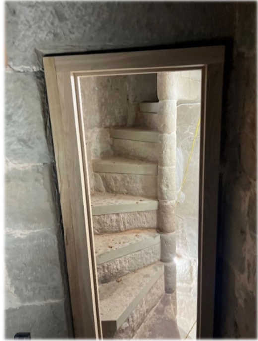
New stair treads and door frame in place.
