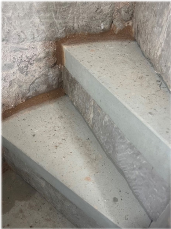
New stair treads fitted
