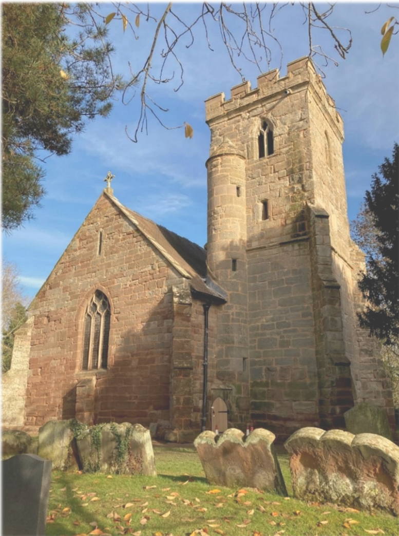
Nave west gable end – stonework pre-project showing cement-base mortar and damp areas.
