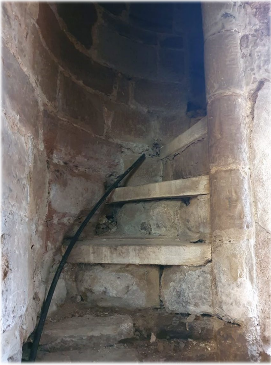
Pre-project: poor condition of internal turret stair treads and pointing.
