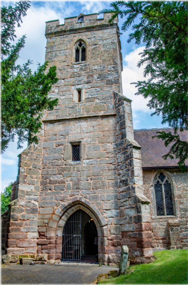
A view of the south tower wall and porch showing the new lime mortar pointing and new window stonework at Level 2. (Image by Droitwich u3a Photography Group).
