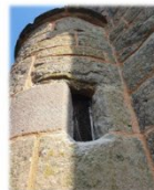
Lime mortar pointing & new stone insert
