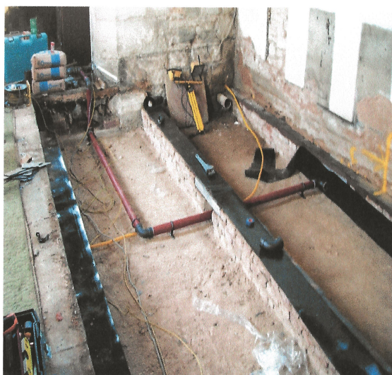
WEEK 1 FOUNDATIONS EXPOSED NEW HEATING PIPES NORTH WEST NAVE
