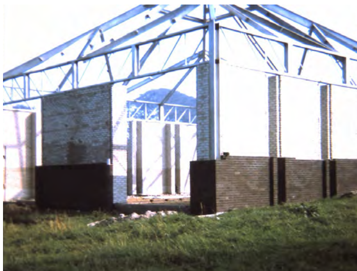
The south west corner
