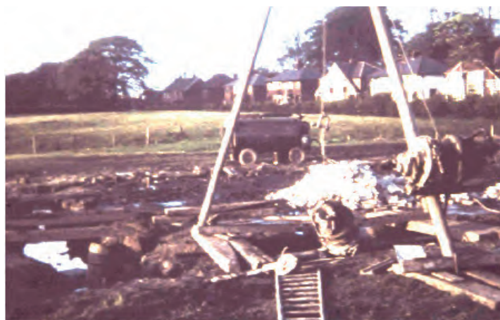
Summer 1969 - work begins on the new church
