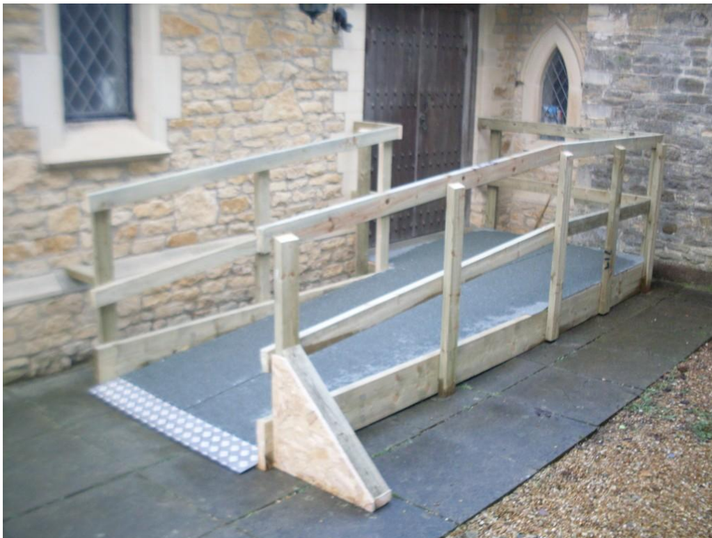
Existing temporary access ramp to be removed
