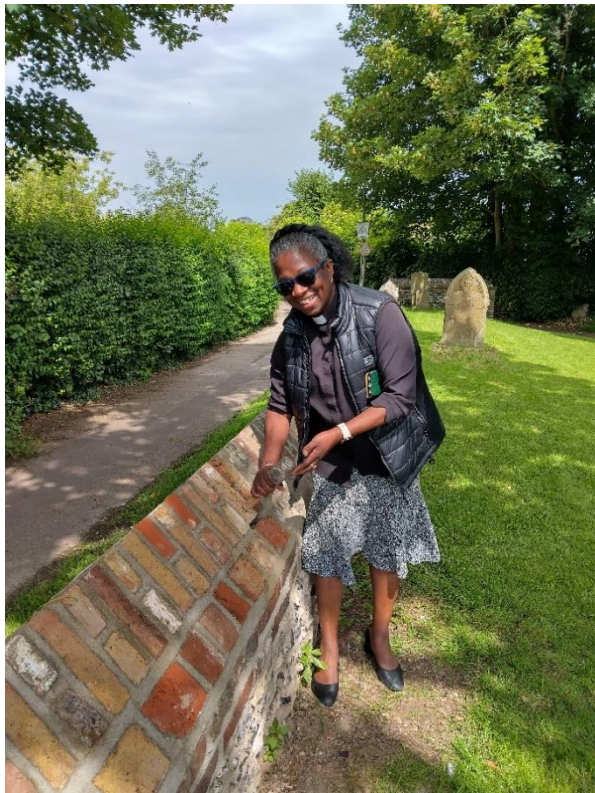
Rev Monica tapping the last brick into place.
