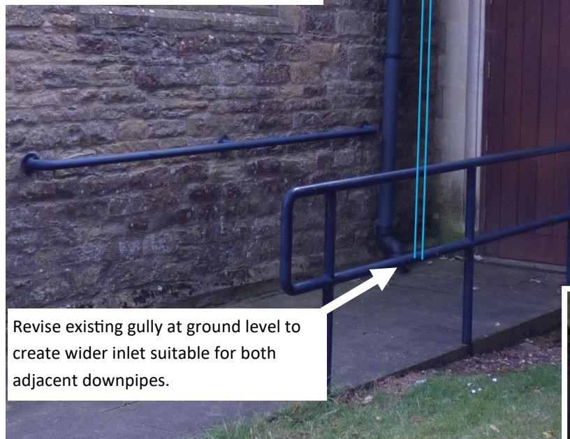
Revise existing gully at ground level to create wider inlet suitable for both adjacent downpipes.
