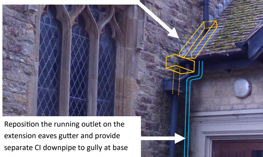
Reposition the running outlet on the extension eaves gutter and provide separate CI downpipe to gully at base
