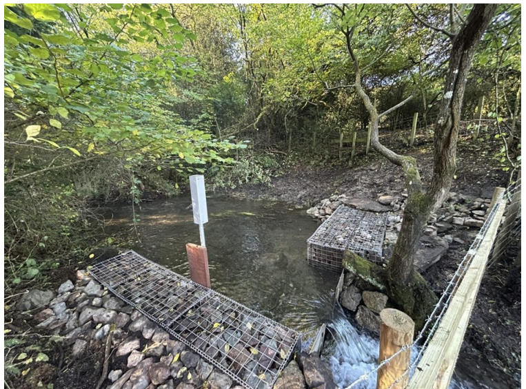
The new flow monitoring structure with telemetry that we installed at nearby Boat Level in 2024.
