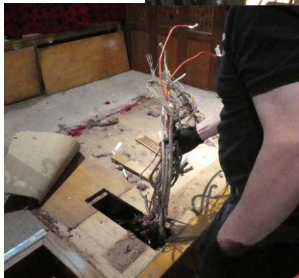
The dubious-looking wiring that connects the console (manuals, stops, pedals) to the pipes
